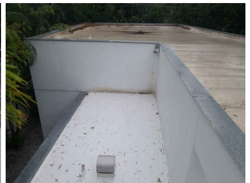
Debris needs to be removed for proper draining.
