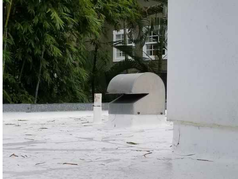
Plumbing vent and exhaust fan vent from bathroom
