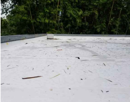
Debris needs to be removed for proper draining.
