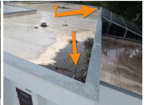
Debris needs to be removed for proper draining.
