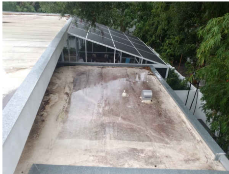
Plumbing vent and exhaust fan vent from bathroom
