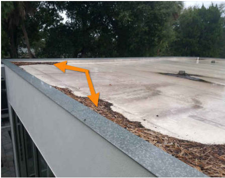
Debris needs to be removed for proper draining.
