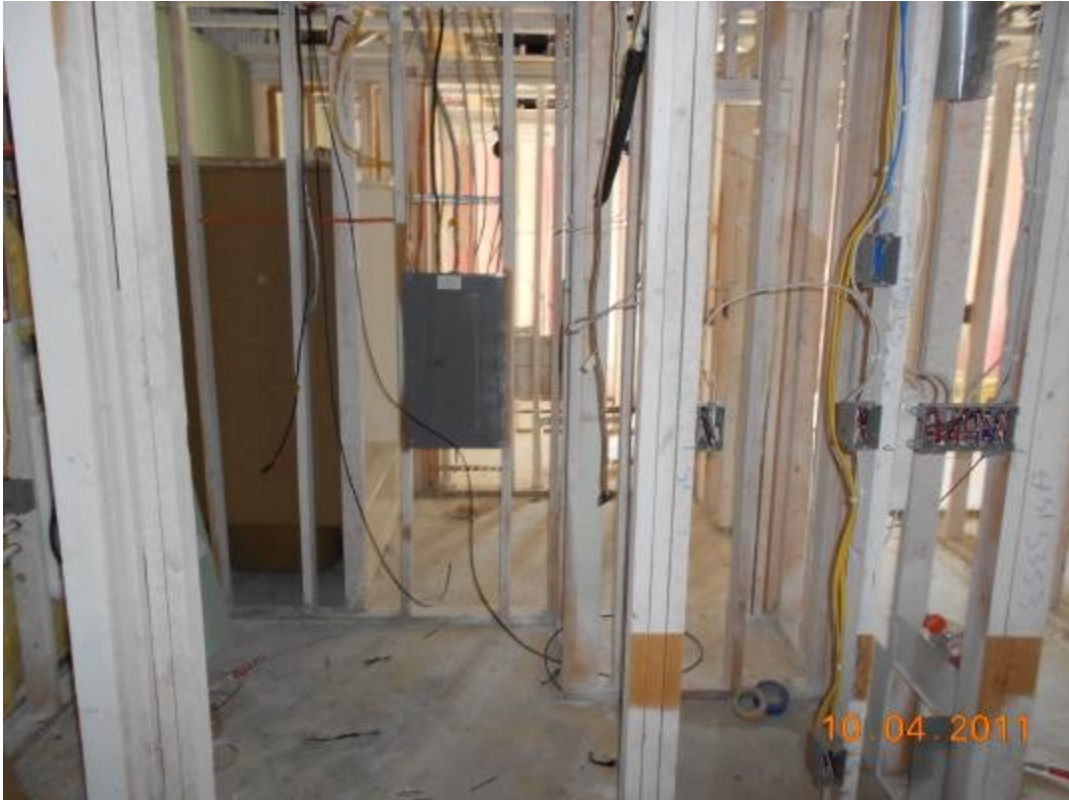
Unit #4 - Carpentry and wiring
