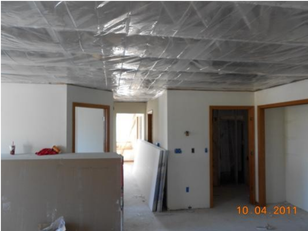
Unit #5 - Vapor Barrier
