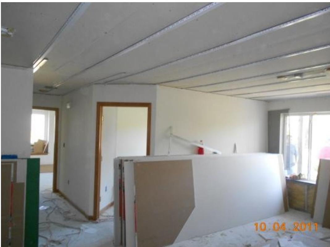
Unit #2 - New ceiling and drywall
