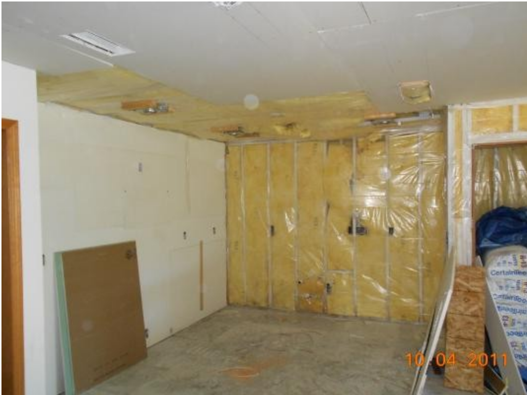
Unit #1 - New drywall and insulation
