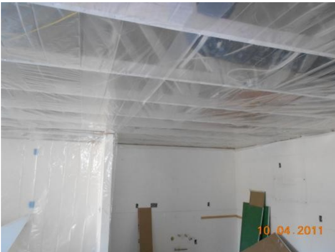
Unit #6 - Vapor Barrier
