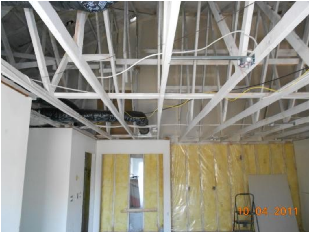
Unit #7 - Carpentry, wiring and insulation
