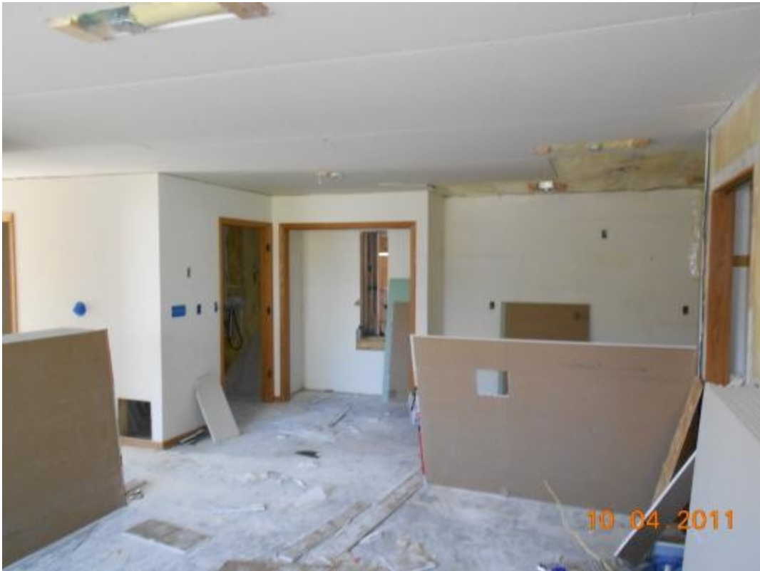
Unit #1 - New ceiling and drywall
