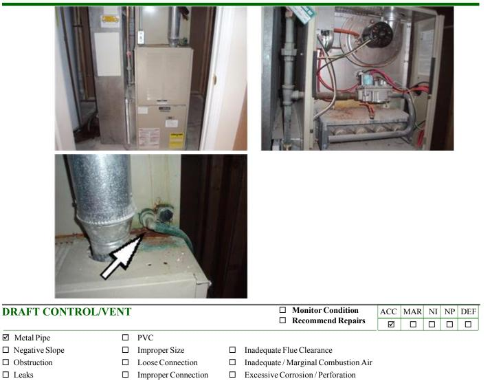
Comments: Metal pipe for furnace and hot water heater are piped into a common flue pipe. Appeared OK at time of inspection.
