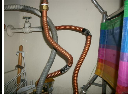
Missing insulation
