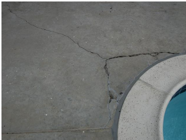
Excessive cracking around pool perimeter
