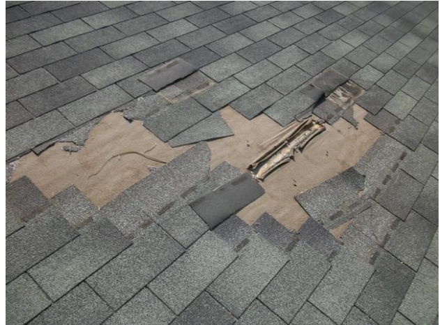
Missing shingles
