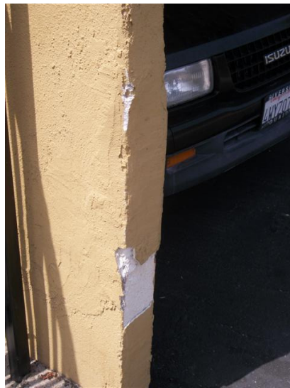
Damaged plaster
