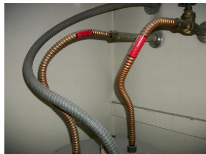
Missing insulation
