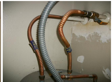
Missing insulation
