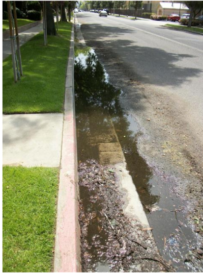
Excessive pooling in front of building
