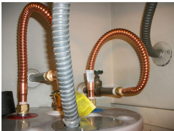
Missing insulation
