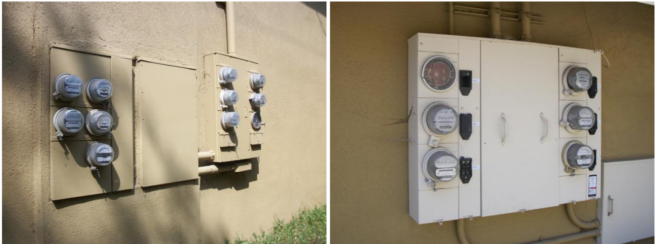
Main panel on right side of building and right side of laundry room
