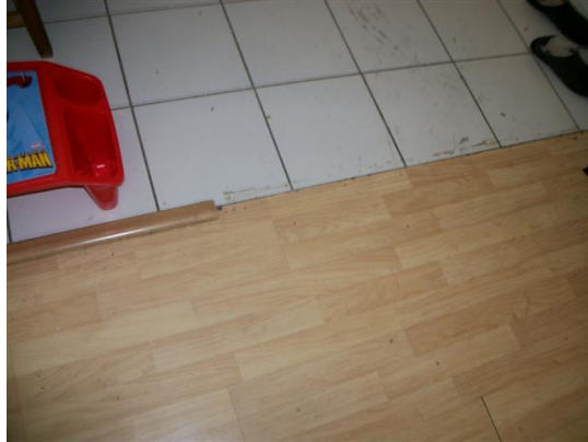
Missing threshold
