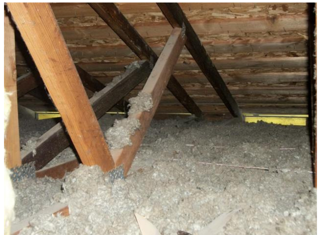
View of insulation
