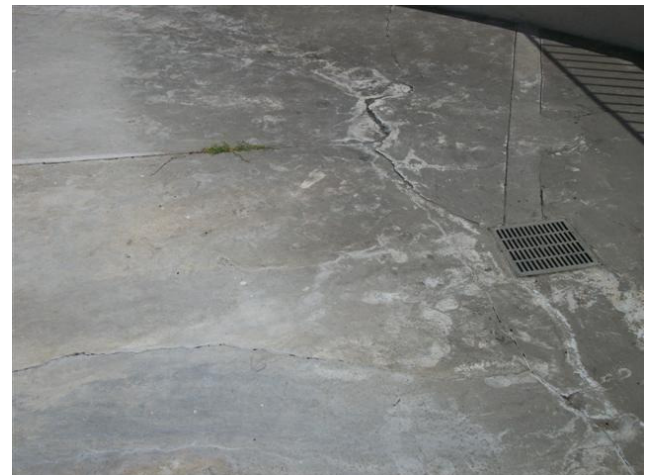
Excessive cracking around pool perimeter
