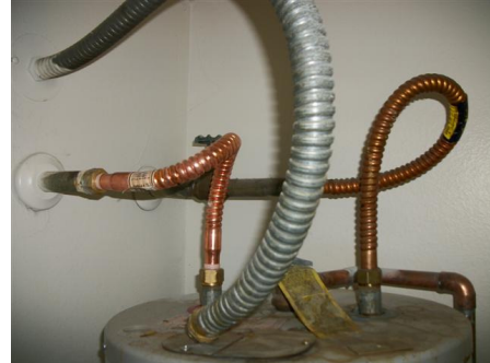
Missing insulation
