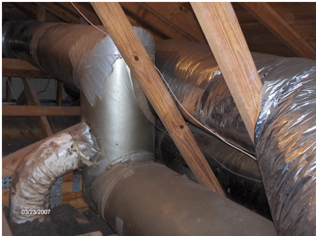
View of ductwork in attic.
