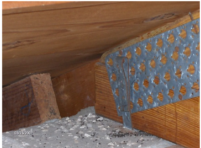
Hurricane strap system present at roof structure.
