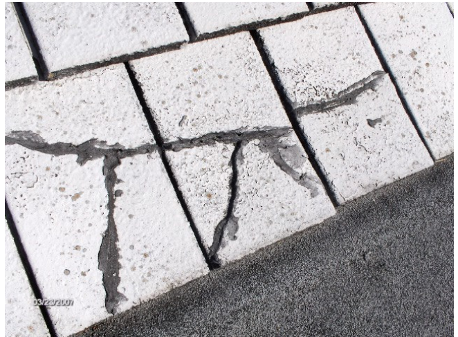
Previous repairs to roof tiles.
