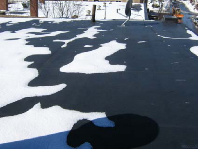
Rubber roof on upper flat roof.
