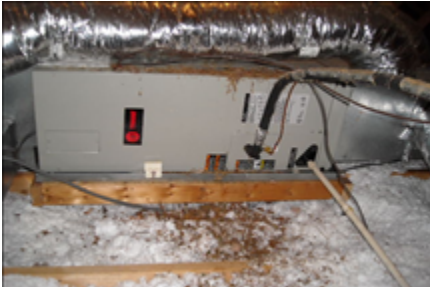
attic insulation is blown fiberglass
