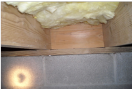
Crawlspace band joist cavities
