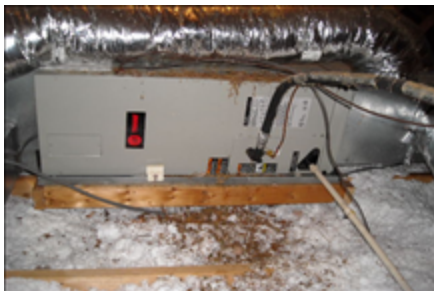
attic insulation is blown fiberglass
